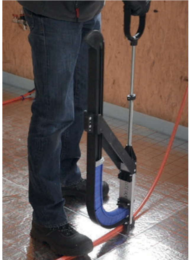
installation with staple system
